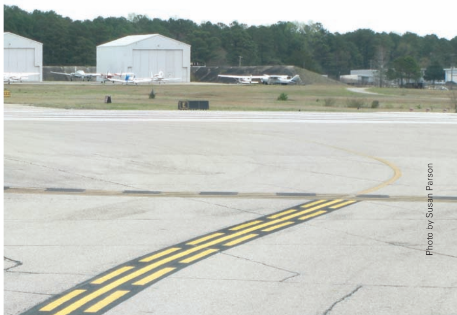
Figure 1. As you can see here, the enhanced taxiway centerlines provide an important warning that you are approaching a holding position marking.
